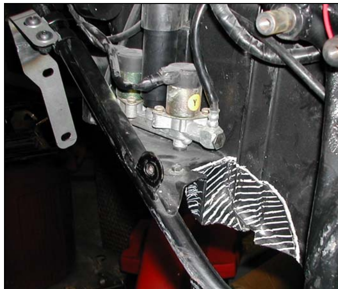
Figure A. Fender Cut Area
